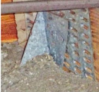
Roof to Wall Attachment:
